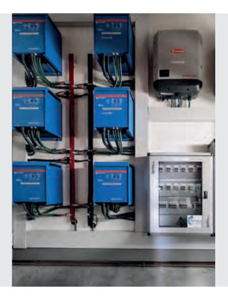
The Fronius inverter provides the MicroGrid with as much PV energy as possible. If the load is less than the maximum capacity of the PV generator and if the batteries are already full (or the charging power of the inverter charger is too low), automatic PV power reduction will be required.
